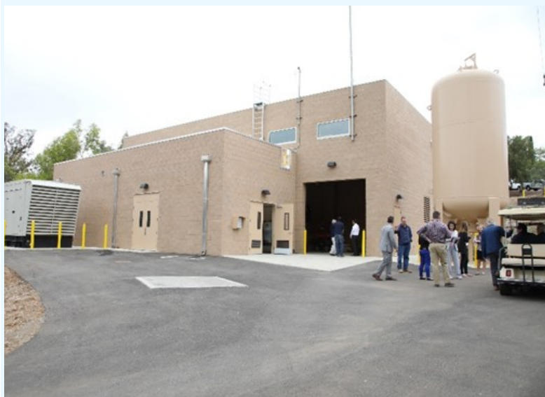
The new pump station at the San Dieguito Dam
